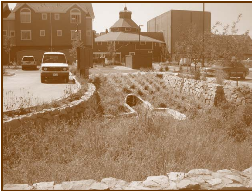
Figure 44: Low Impact Development Principles, Storm-water management using natural plantings to filtrate water run-off.
